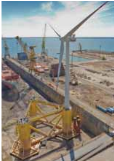
1) Construction 100% on shore
